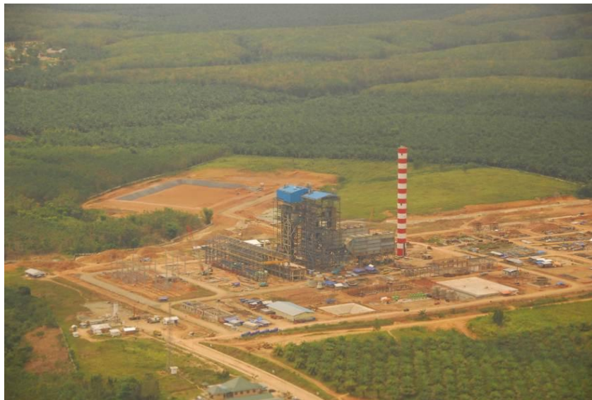
An aerial view of 2X30 MW mine-mouth power plant construction site
