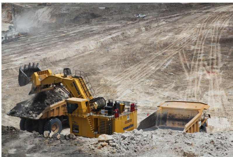
New heavy equipment operated by SIS: double side loading, 400 tonne hydraulic excavator PC4000, loading two 200 tonne Caterpillar 789, overburden trucks
