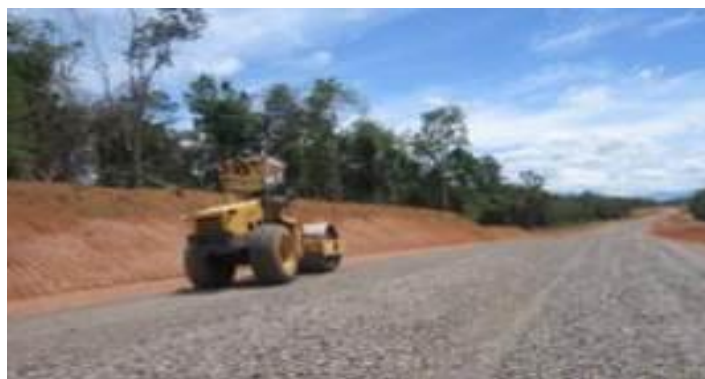
Haul road construction at Balangan.
