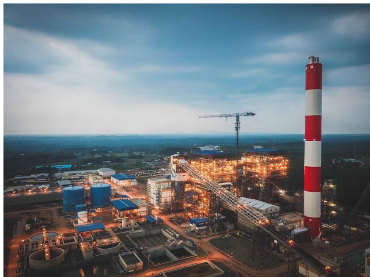
PT Tanjung Power Indonesia's 2x100 MW power plant in Tanjung, South Kalimantan.
