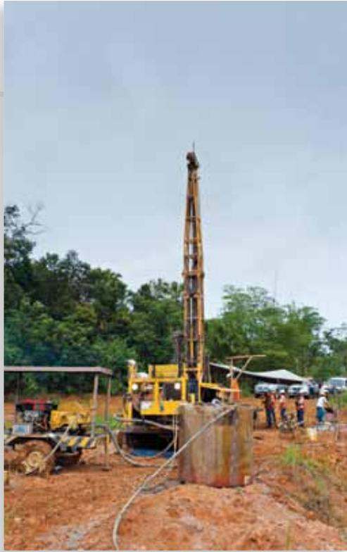
Geotechnical core drilling was conducted in Wara 1, North Paringin and Tutupan pits.
